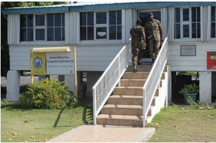
Service members entering the recently renovated JDF Credit Union building
